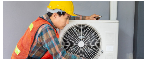
Technician installs a residential heat pump
