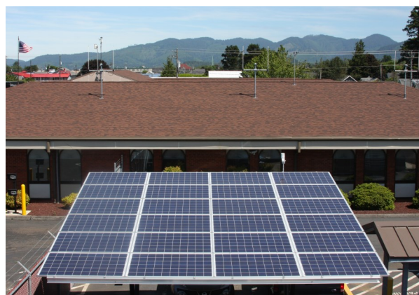
Tillamook PUD's headquarters has solar on site.
