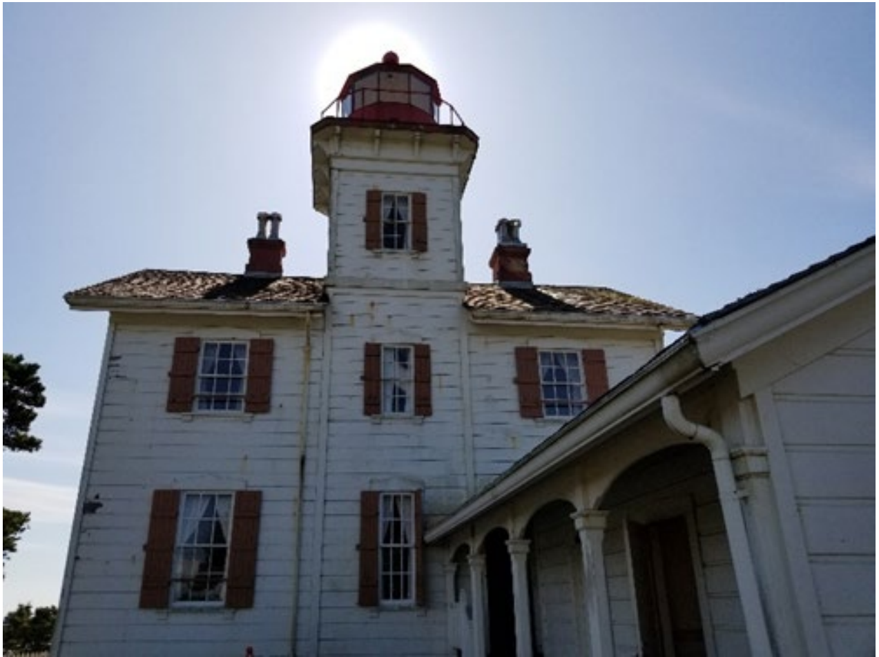
Figure A.1 – Exterior
